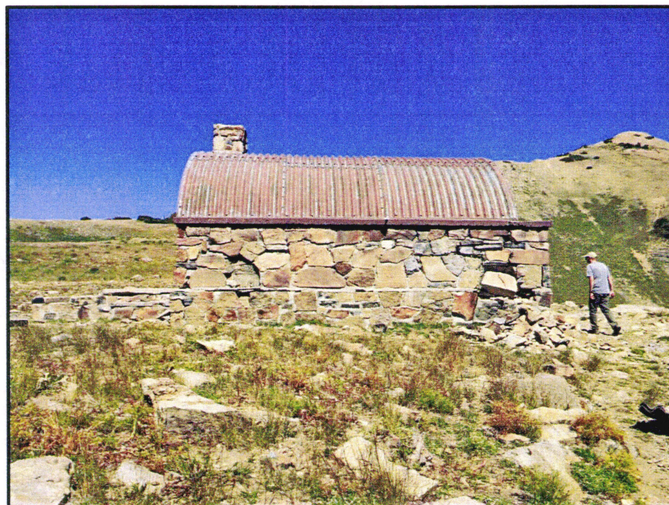
Back and south facing side.
